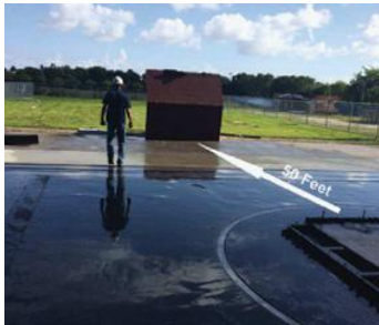
Figure 14: Test house rolled 50 feet away after foundation failure.
