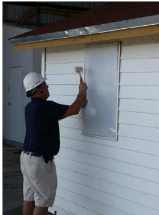
Figure 5: Installation of Storm Stoppers Original 3/8 in. on rear window.
